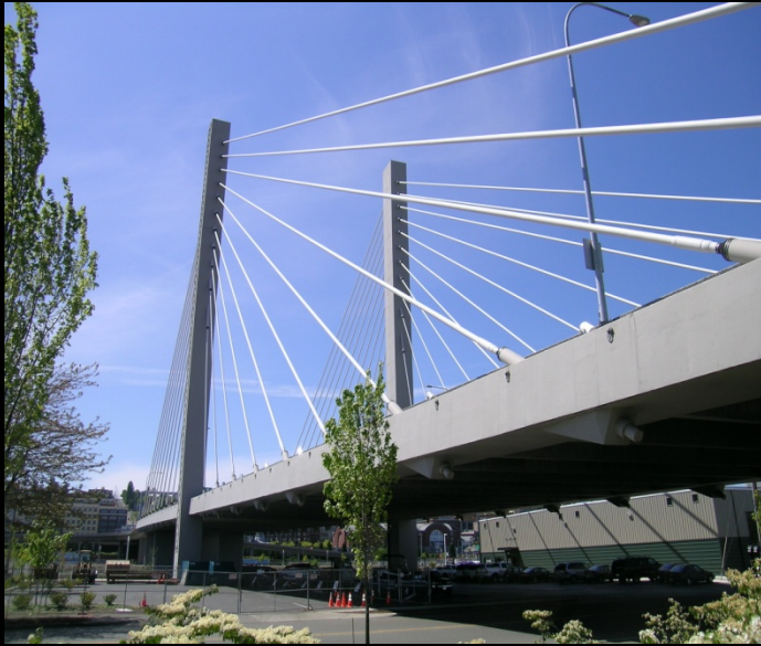
Foss Waterway Cable Stay,
